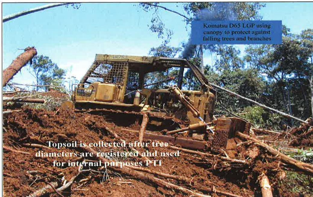
Figure 4-21: Topsoil Removal (Photo PTI)
